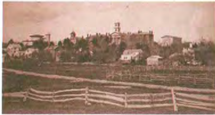
Fig. 5. Amherst College row with Johnson Hall in center (Archives and Special Collections, Amherst College)
