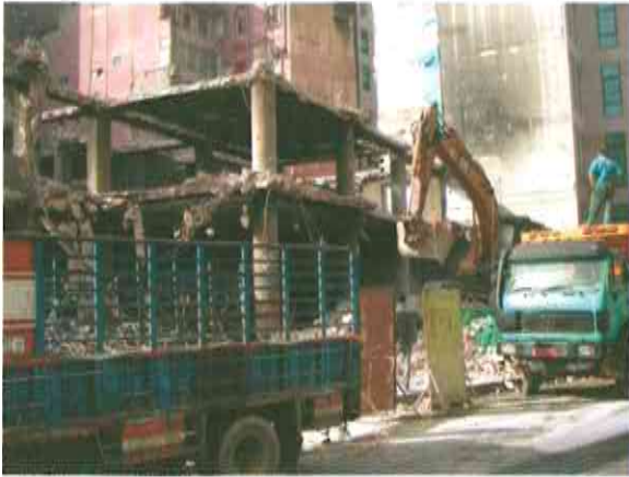
Fig. 12. Demolition of low-rise apartment building, Bliss Street, 2007 (Photograph by the author)
