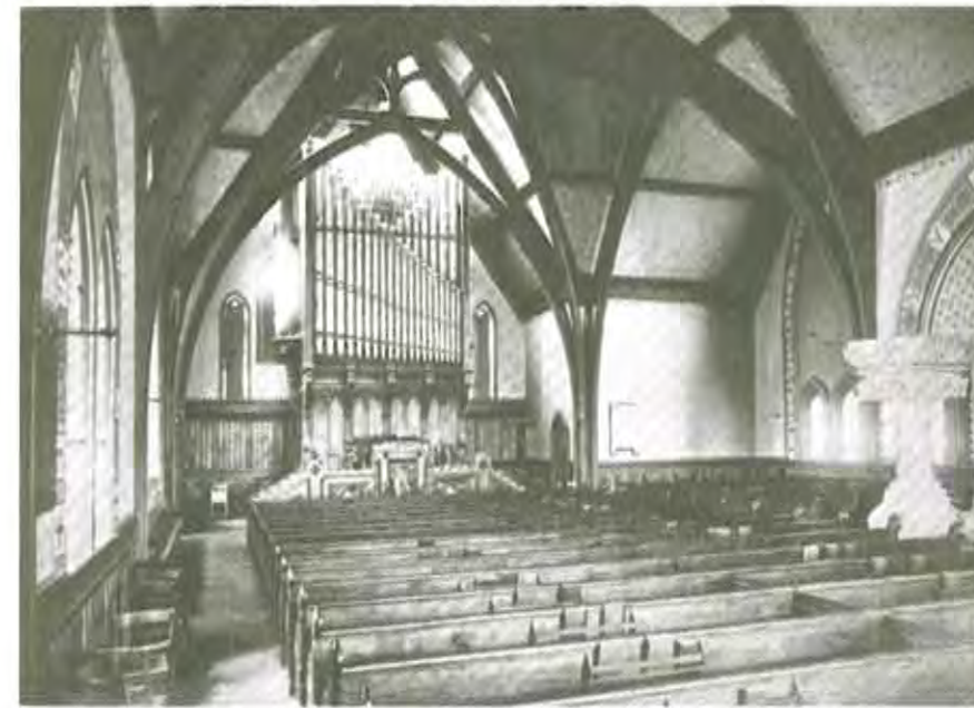
Fig. 12. Two views of Amherst College Stearns Church, interior (Archives and Special Collections, Amherst College)
