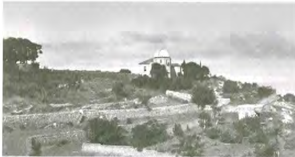
Fig. 5. Inspired by traditional rural practices, stone wall terraces were constructed along the length of the campus escarpment to rehabilitate the rocky slopes and enable planting. (AUB Department of Photography, The Moore Collection)
