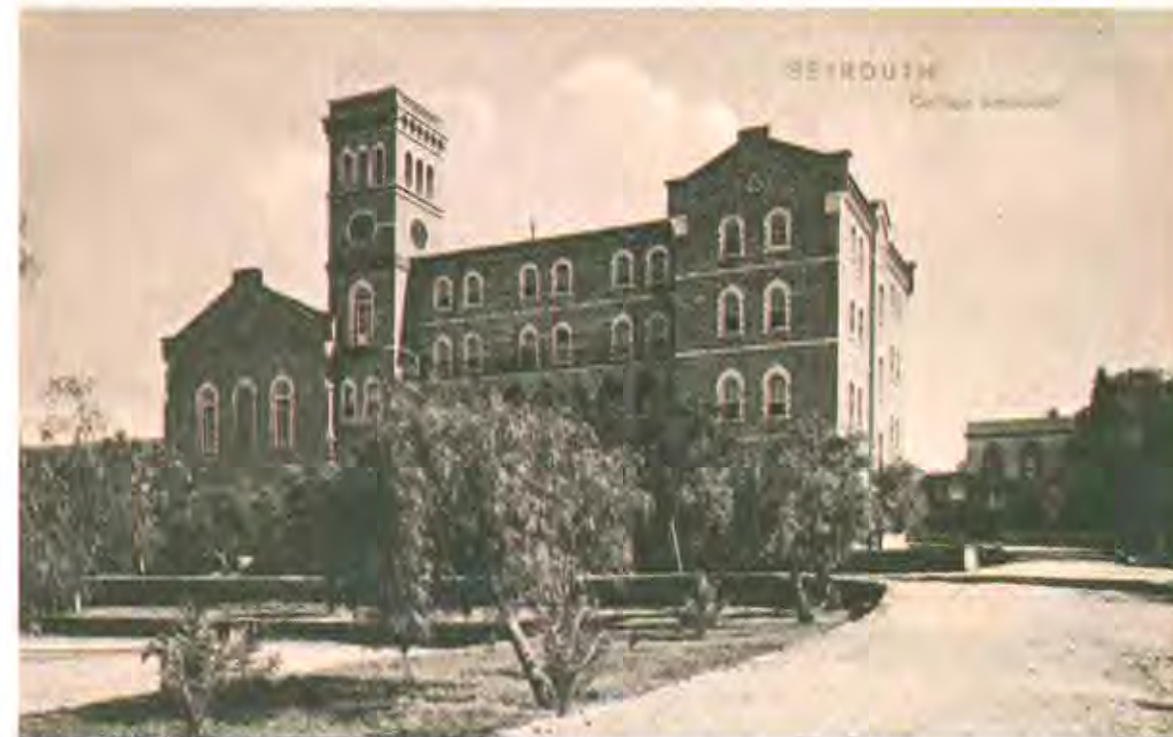
Fig. 2. College Hall, south façade (Photo courtesy of Camille Tarazi)
